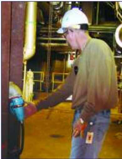
Mechanics can quickly and safely make and break electrical connections, without special PPE.
