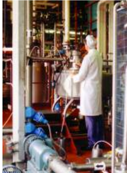
Electrical connections production area - chocolate factory
