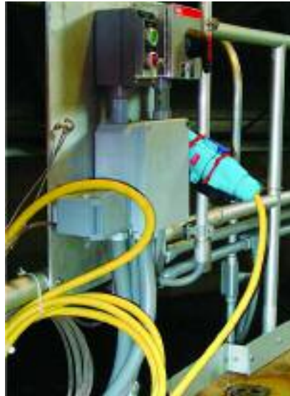
Wastewater Mixer Connection
