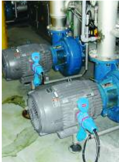
Process Pump Connections
