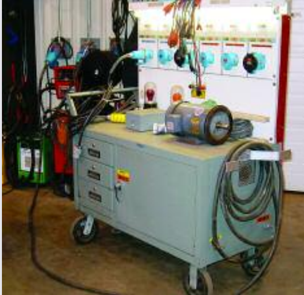
Correct motor rotation can be ensured by pre-testing motors at a test bench with receptacles that match the polarization in the field.
