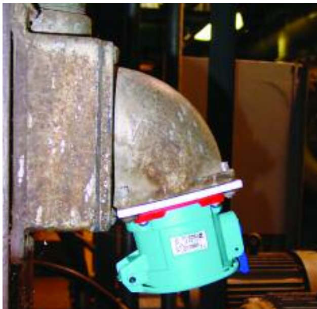
Adapter plates made it simple for this power plant to convert their existing pin and sleeve receptacles to Deconnectors.
