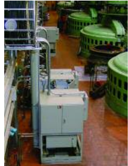
Power Receptacles (lower left)
