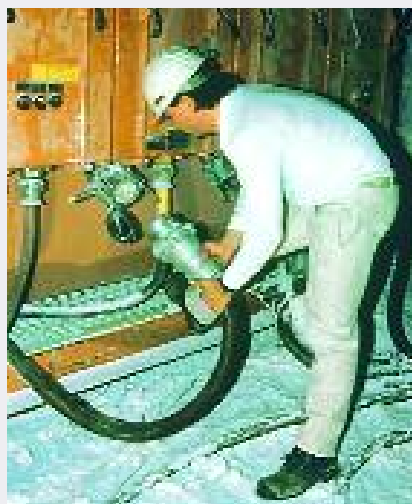
Mobile generator at salt mine
