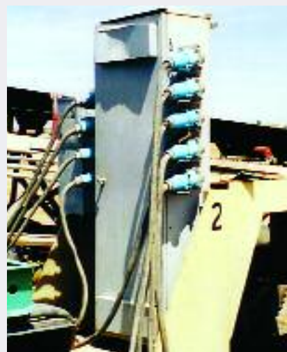
Mobile power distribution panel
