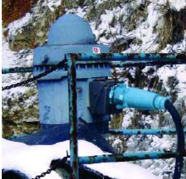
A 200A, NEMA 3R rated DS Series DECONTACTOR connects power to a float pump via a direct mounting configuration. When required, the DS receptacle is disconnected and the pump is easily relocated to another retention pond.
