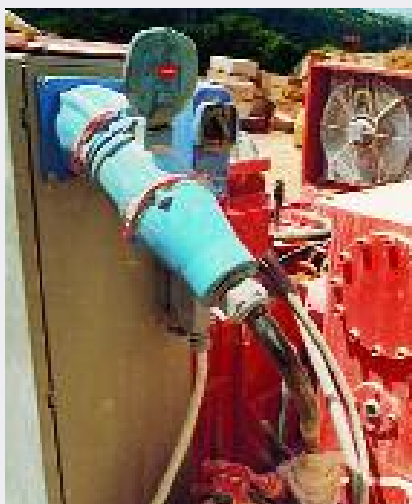
Power connections to a marble cutter
