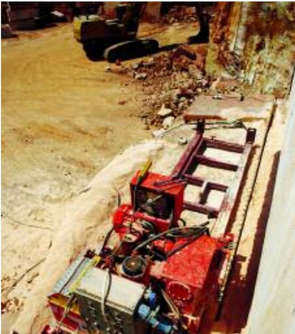
Meltric DS devices supply power to large cutting machines at a marble quarry. DS's are UL and CSA switch rated, allowing them to function as a 'line of sight' disconnect.
